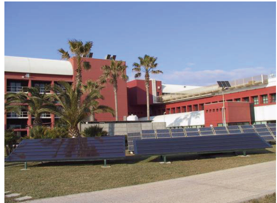
Figure 1: Plant site installation in Portici (NA)
