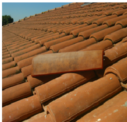
Figure 1: The indistinguishable PV TILE just in the middle of a roof
